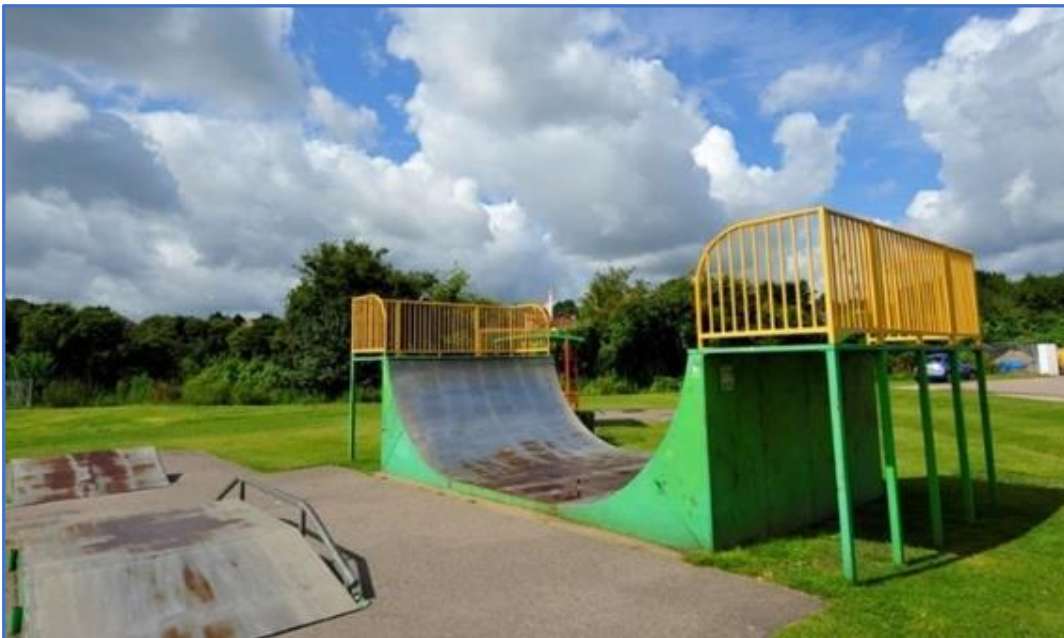
Figure 1: The existing ramps and half-pipe at Mill Meadow: steep, short, narrow and noisy – a barrier to participation
